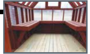
Treated Wood Floor/ Planting Shelves
